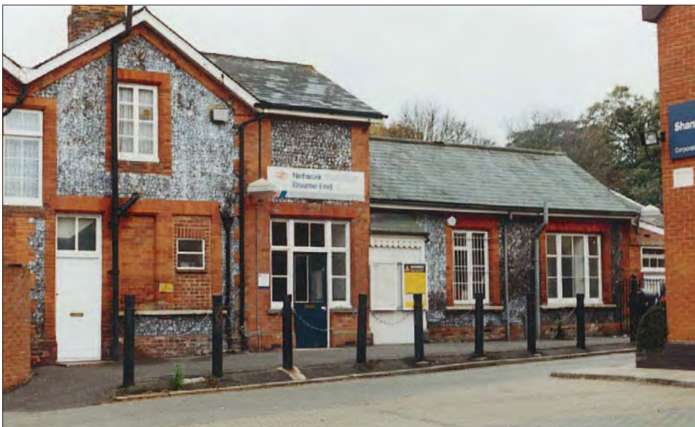
Left: the street facade of Bourne End station displays the local flint-and-brick construction style. On the left is the station master's house, and at extreme right is the modern building which has covered the site of the bay platform run-round loop.
