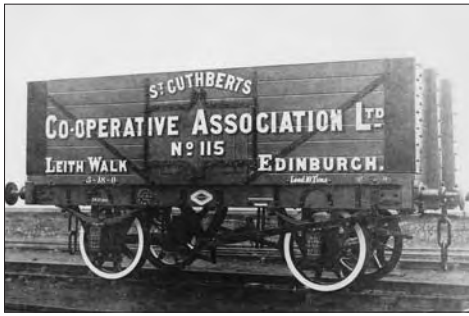
St. Cuthberts Co-operative Association Ltd. No.115 – this is a 10-ton mineral wagon built by R. Y. Pickering & Co. of Wishaw in 1905. It is a side door wagon, but the doors are cupboard style which was a feature of many wagons used in Scotland. It is also fitted with a non-standard brake. There is a semi circular plate over the brake handle indicating 'off' and 'on'. About this time there was much experimentation with new 'patent' brakes. Photograph: HMRS Peter Matthews Collection.
